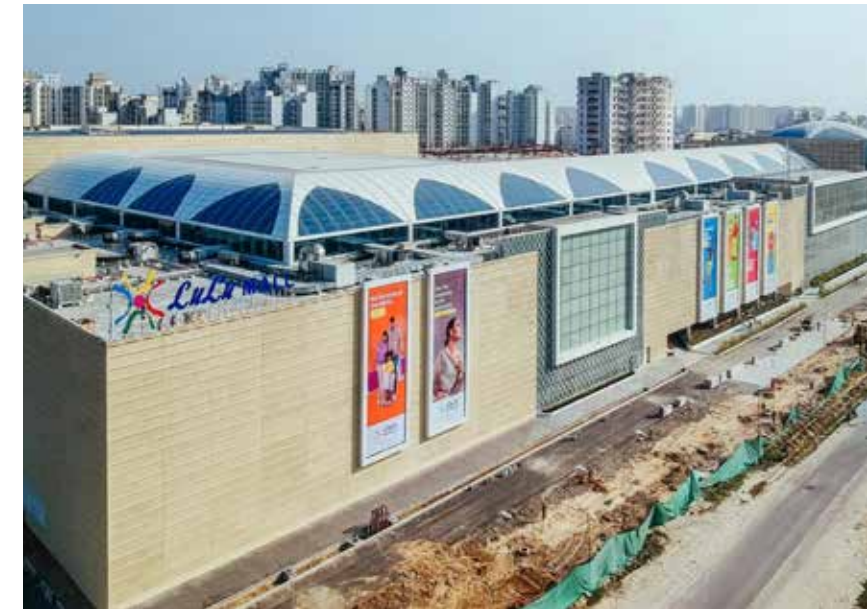
Lulu Mall, Lucknow
